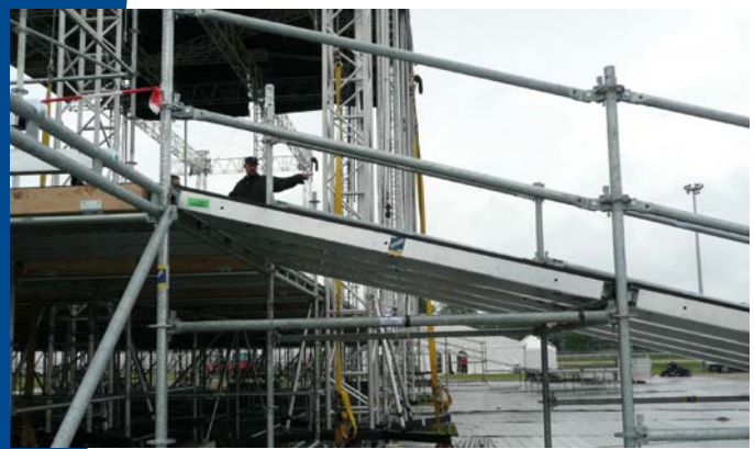
Thanks to the flexibility of the MP system, it is also possible to create stage walkways and access ramps of any size.
